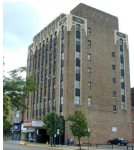
The Hooker-Fulton building in Bradford, PA, the site of first Ryder Scott office in 1930s, was visited by Don May in June.
